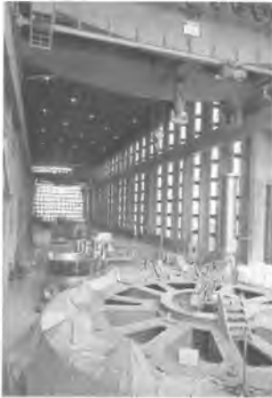
Figure 8 Interior of the turbine hall in Đerdap HPP under construction. KONČAR delivered three 190 MVA hydrogenerators, 1240 tons each, which were put into service in 1972.
