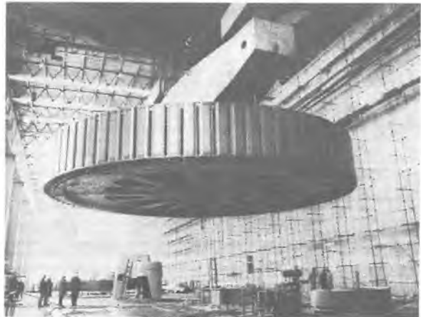
Figure 8 Interior of the turbine hall in Đerdap HPP under construction. KONČAR delivered three 190 MVA hydrogenerators, 1240 tons each, which were put into service in 1972.
