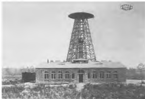
Fig.7 Long Island Plant
