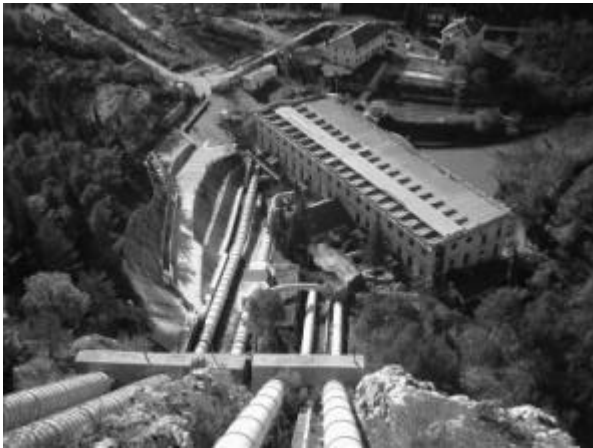
Fig. 9. Penstocks, bifurcation and powerhouse
