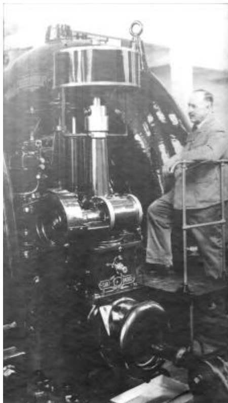
Fig. 2. Original turbine governor
