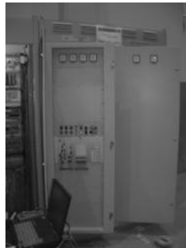
Fig. 7. Digital voltage regulator of G 2
